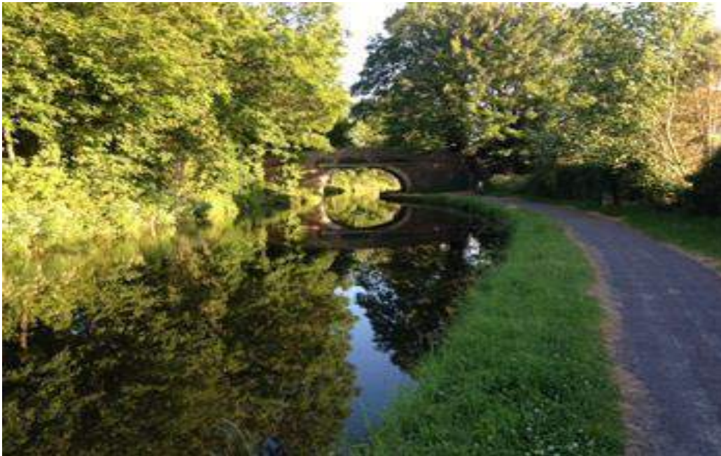
Photo 4. Hatlex Bridge (No. 119) on Lancaster Canal
