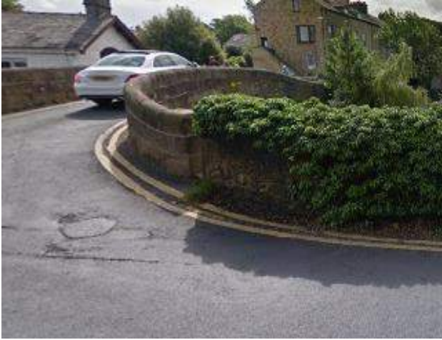
Photo 33. Canal Bridge on Hest Bank Lane
