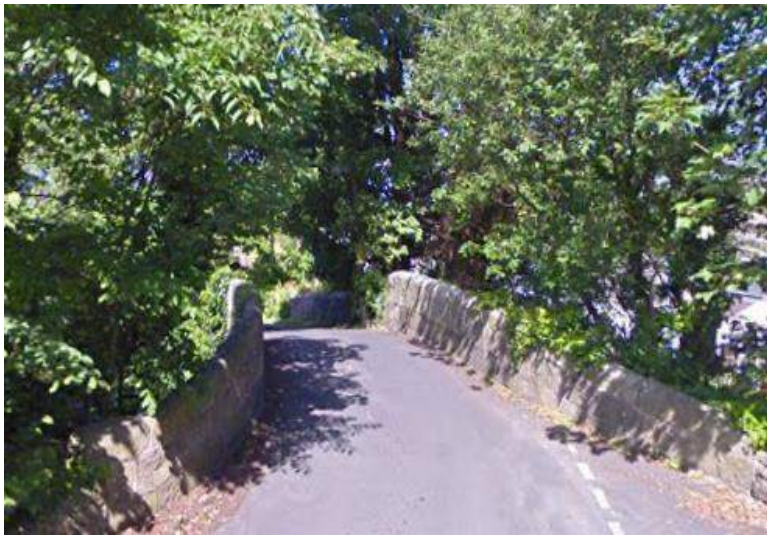
Photo 34. Canal Bridge on Hatlex
