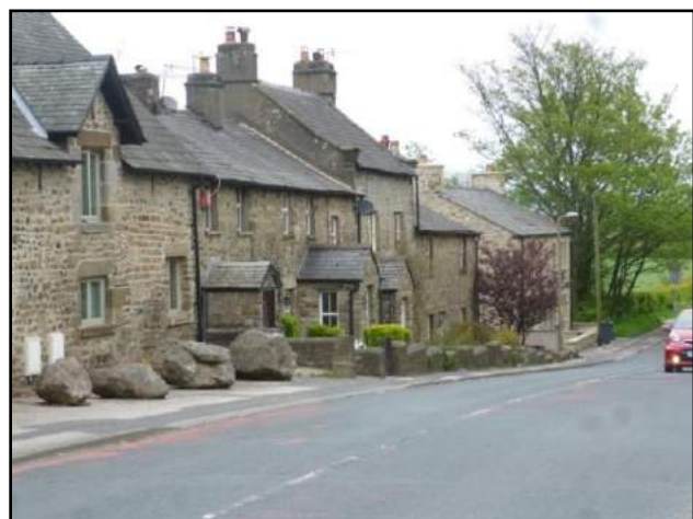
Photo 6. Stone Cottage, Main Road, Slyne
