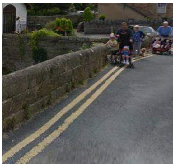
Photo 37. Pedestrians on Hest Bank Lane Canal Bridge
